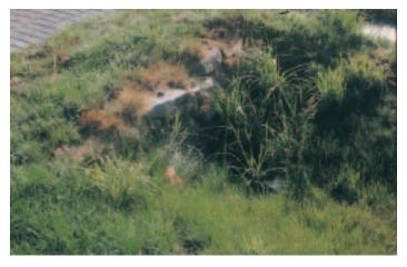
Figure 3. Grass swales rather than curb and gutters enable water to infiltrate and reduce the erosive effects from rapid discharges into streams.
