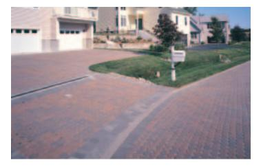
Figure 2. Slot drains at the ends of the PICP driveways facilitated sampling and collection of runoff.
